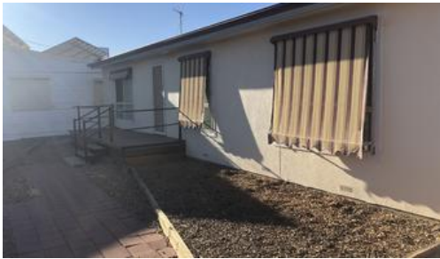
519 Chapple Lane, Broken Hill
